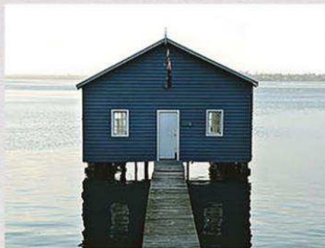
BOATHOUSE & DOCK REPAIR
