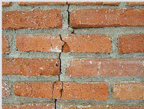
PIER & FOUNDATION REPAIR
